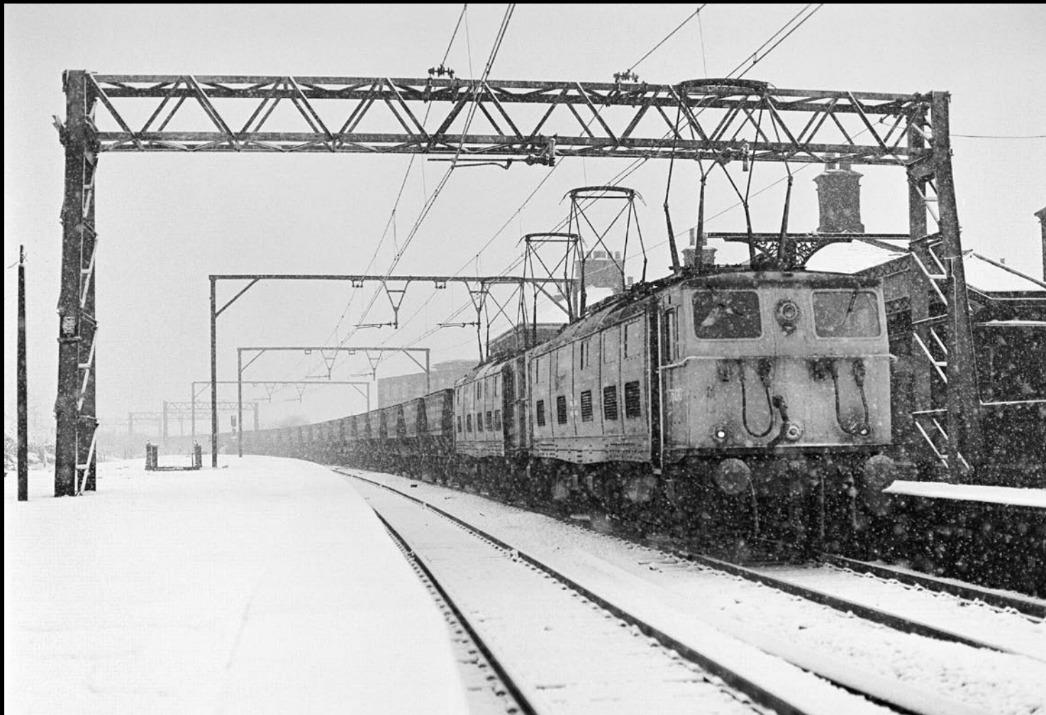
Below: The amazing Woodhead route with its 1,500V dc overhead electrified network always roused some interest with photographers. During a blizzard on 31 January 1980, Class 76s Nos. 76026 and 76010 pass through Penistone station with a Merry-go-Round (MGR) coal service. Soon after this picture was taken much of the surrounding area was impassable to both road and rail traffic. Colin J. Marsden Photographic details: Camera: Mamiya 645 1000S, Lens: Mamiya 80mm, TriX at 400ASA, Exposure: 1/500 @ f5.6. Negative scanned on Nikon Coolscan9000 at 600dpi.
