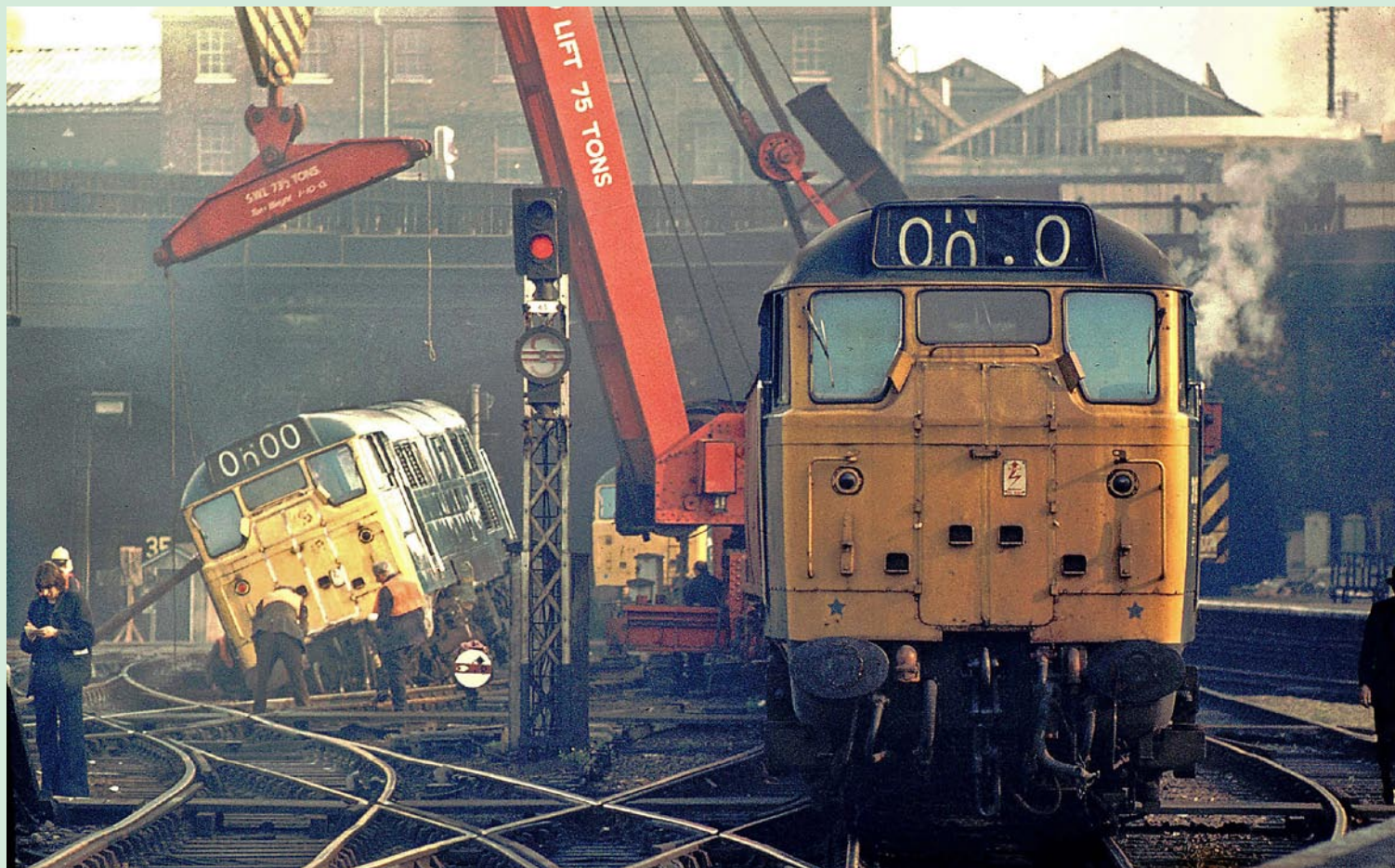
Below: Trouble at London King’s Cross, on 10 May 1976 Class 31 No. 31174 became derailed at the entrance of the station during a light loco move between the loco yard and platforms. The problem caused chaos to station workings for hours and here the rerailing operation is performed by a steam crane. Charlie Robbins Photographic details: Not supplied
