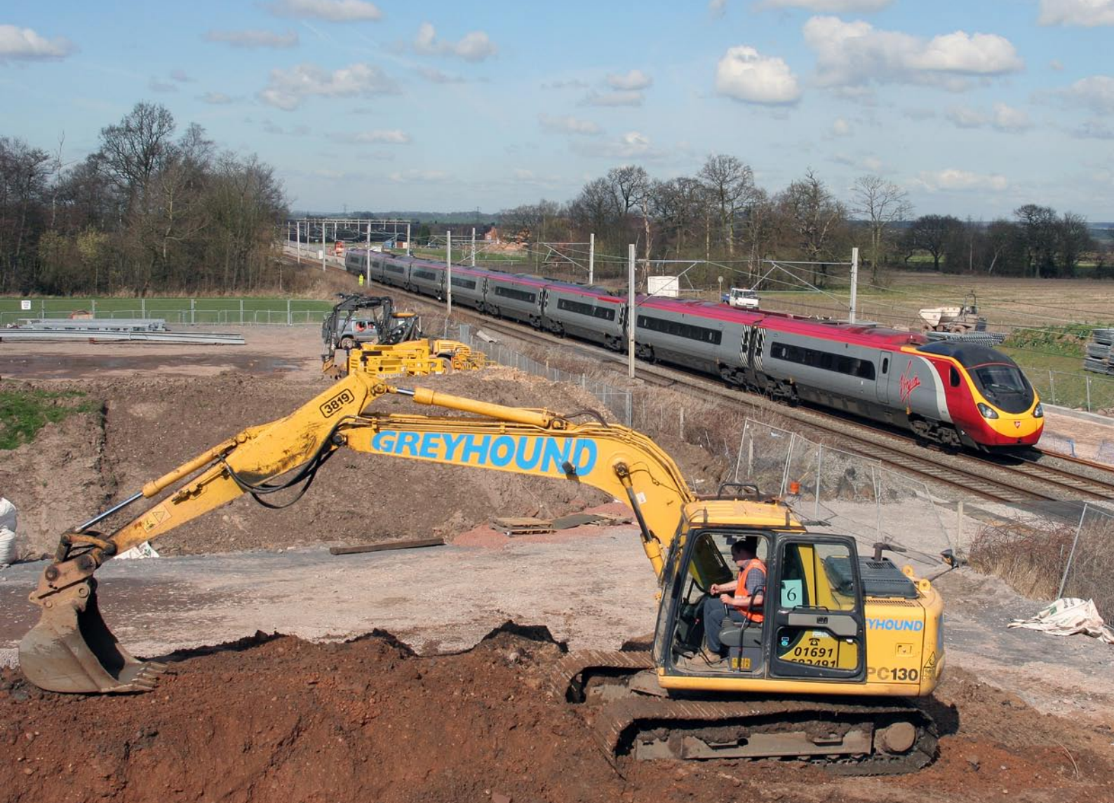
Above: Work continues to widen the Trent Valley section of the West Coast Main Line (WCML) north of Tamworth. This was the scene at a location called Hanch on 21 March 2007 with work progressing adjacent to the line. A Pendolino travels south at high speed passing ongoing groundworks for forthcoming quadrupling of this section, a major Network Rail operation but one which will see capacity of the Rugby-Stafford section of the route considerably increase. Tom Curtis Photographic details: Camera: Canon EOS350D, Lens: Canon 28-105mm zoom at 28mm, ISO: 400, Exposure: 1/1000 @ f9
